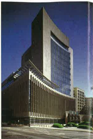
The design of the Federal Courthouse constructed in the mid-1990s in downtown Minneapolis betrays neither its space and budget constraints nor the extensive security requirements the building had to meet.
